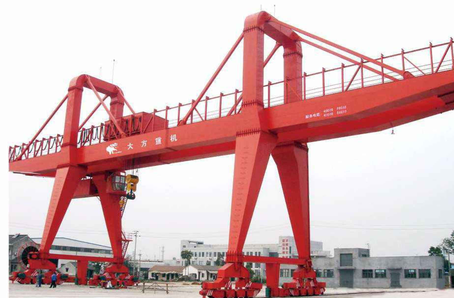
装卸桥 loading bridge
