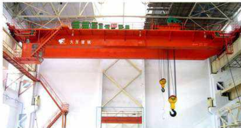
QB 型防爆桥式起重机 QB explosion-proof overhead crane
